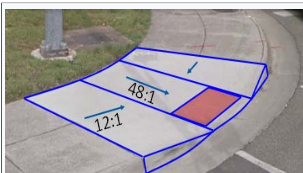
This is an example of a CG-12 type A curb ramp installed on Elm Avenue in the City of Roanoke Google Maps Link
